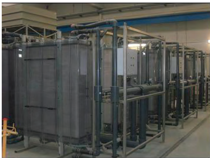
Fig. 4. EDR stacks at the Depurbaix WWTP.
