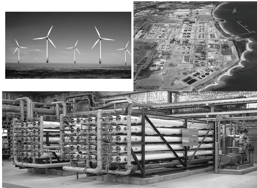
Fig. 8. The Kwinana Seawater Reverse Osmosis Desalination (SWRO) Plant and Wind Farm in Perth, Western Australia . 8a ( Upper Left ) The SWRO Plant seaside location in Pert; 4b ( Upper Right ) The Emu Downs Wind Farm consisting of 48 Vestas wind turbines each with 1.65 MW generating capacity; 4c ( Lower ) The desalination plant, with 12 SWRO trains with a capacity of 160 megalitres per day and six BWRO trains delivering a final product of 144 megalitres per day. (Pankratz, 2008).
